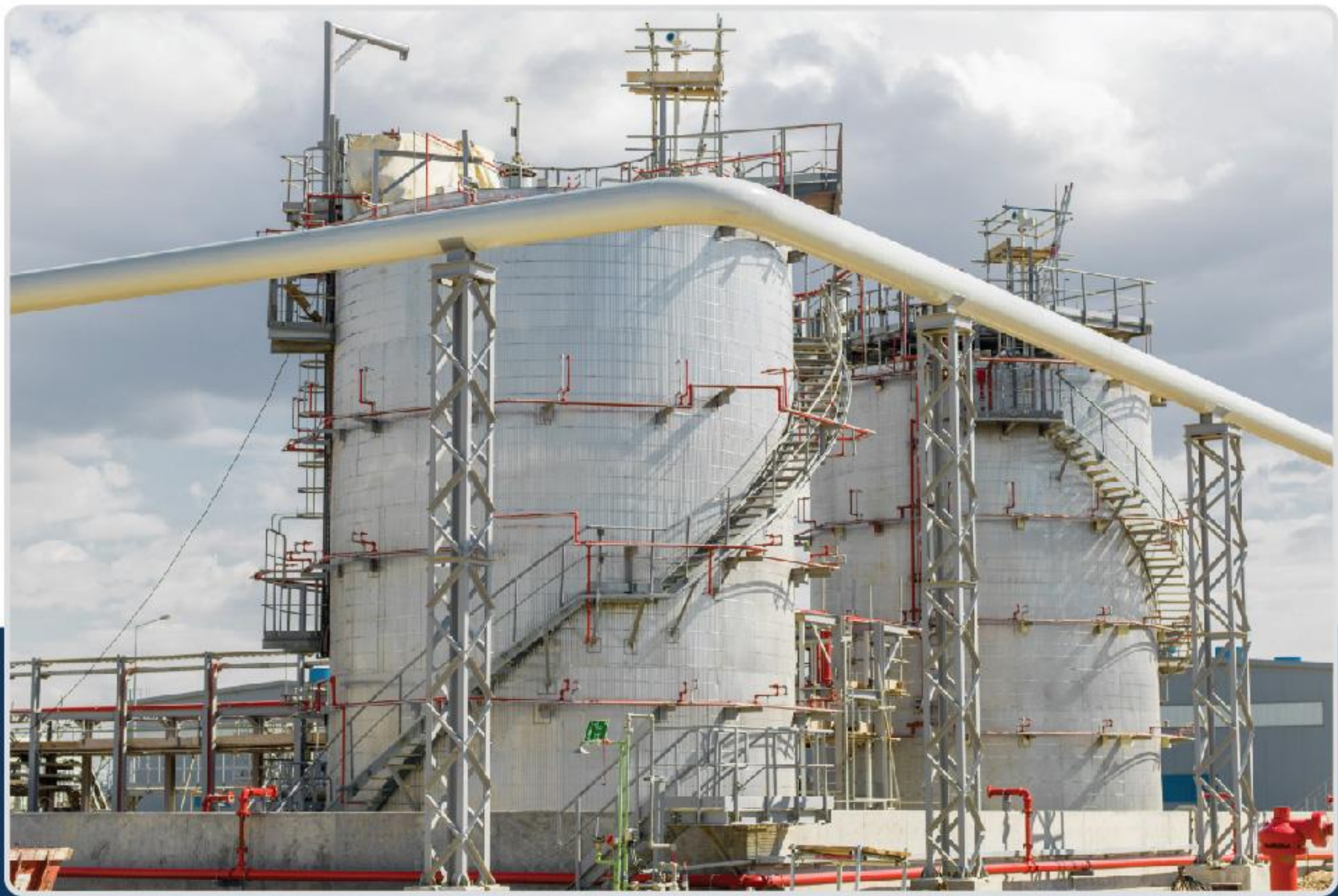
GOSP (Gas & Oil Separation Plant)
